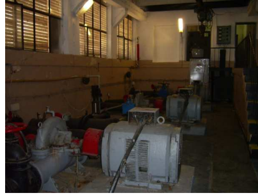
Figure: PS Mokrishte – II uplift – pumps high pressure
