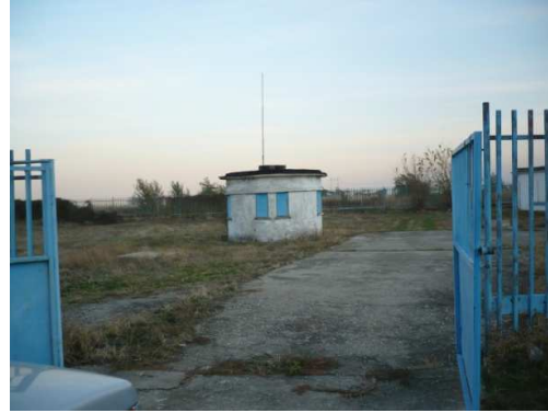
Figure: Varvara – Vetren dol water yielding zone - LJK
