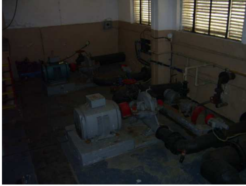
Figure: PS Mokrishte – II uplift – pumps low pressure
