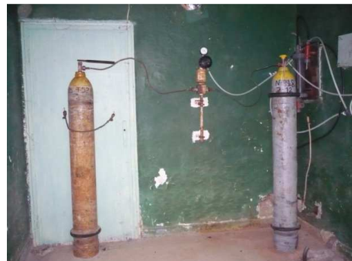
Figure 3-19 Figure 3 18 Disinfection with chlorine gas in the chlorination station next to Vetren PS – II lift
