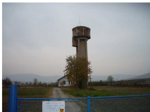
Figure 3-24 Water tower of V=20m^3 for the village of Sinitevo
