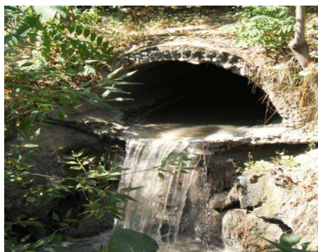
Figure 3-36 Outfall of drainage canal of Collector
