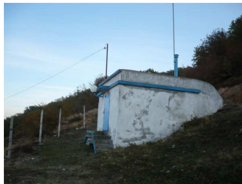
Figure 3-32 PR of V=500\text{ m}^3 – high zone for the village of Simeonovets
