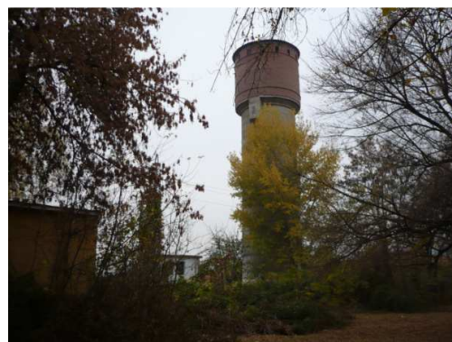
Figure 3-25 Water tower of V=250m^3 for the village of Ognyanovo
