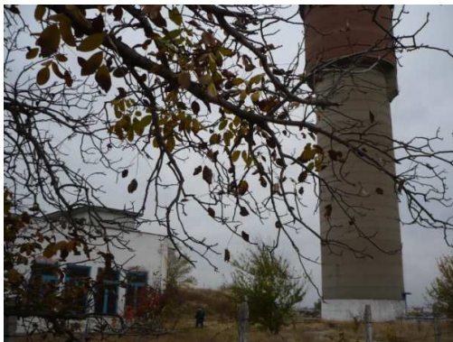
Figure 3-29 Water tower of V=250\text{m}^3 for the town of Septemvri
