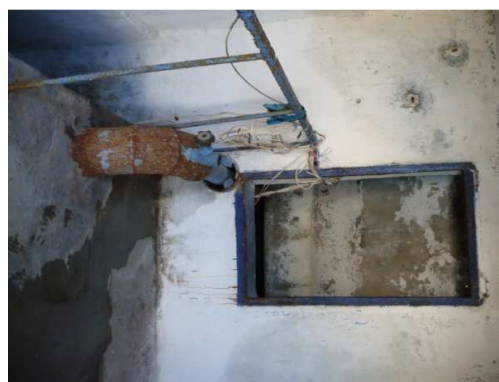
Figure 3-33 Suction tank of V=25\text{m}^3 of Semchinovo-Simeonovets PS
