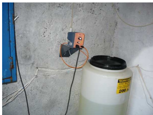
Figure 3-20 Disinfection with sodium hypochlorite in PR of V=500 m 3 – high zone for the village of Simeonovets
