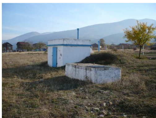
Figure 3-33 Suction tank of V=25\text{m}^3 of Semchinovo-Simeonovets PS
