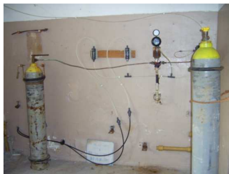
Figure 3-12 Disinfection with chlorine gas in Mokrishte PS - II lift
