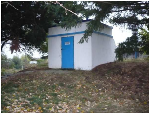
Figure 3-27 Suction tank of V=50\text{m}^3 of Vetren PS – III lift
